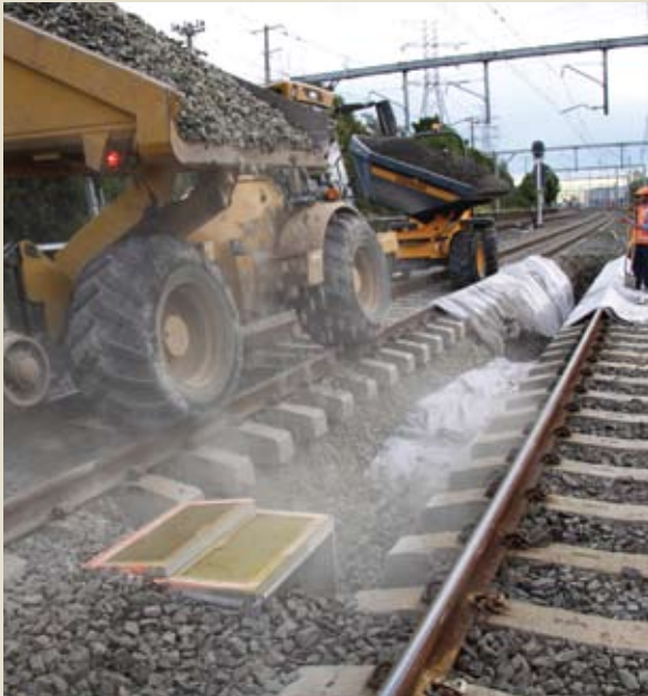
HardieAquifer™ concrete pipes in action on a NSW rail project.
